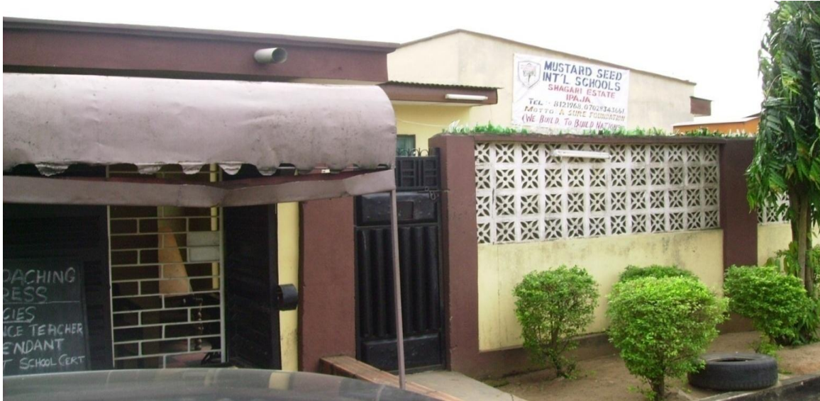
Plate6.4: One of the three bedroom houses that Was Fenced And Converted/Transformed to a school
