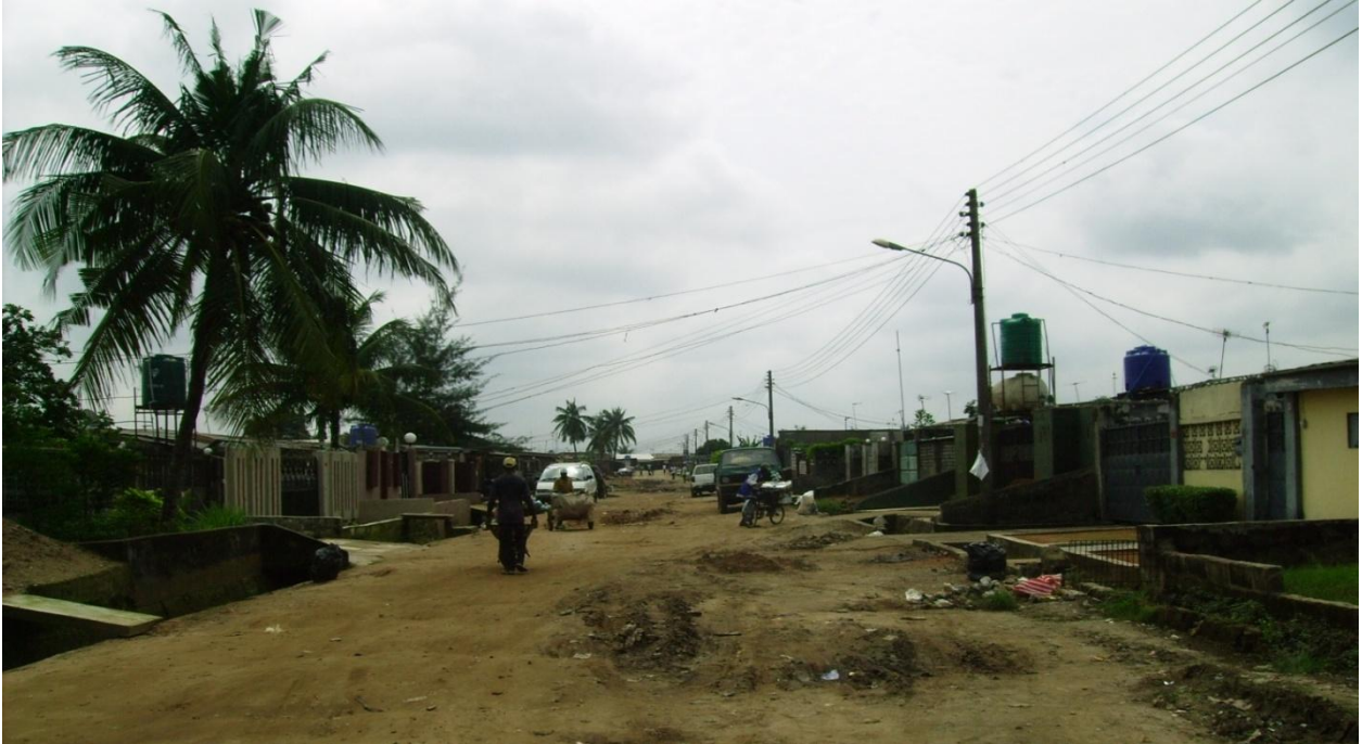
Plate 7.2: showing one of the numerous bad roads due to excessive pressure of traffic within the Estate
