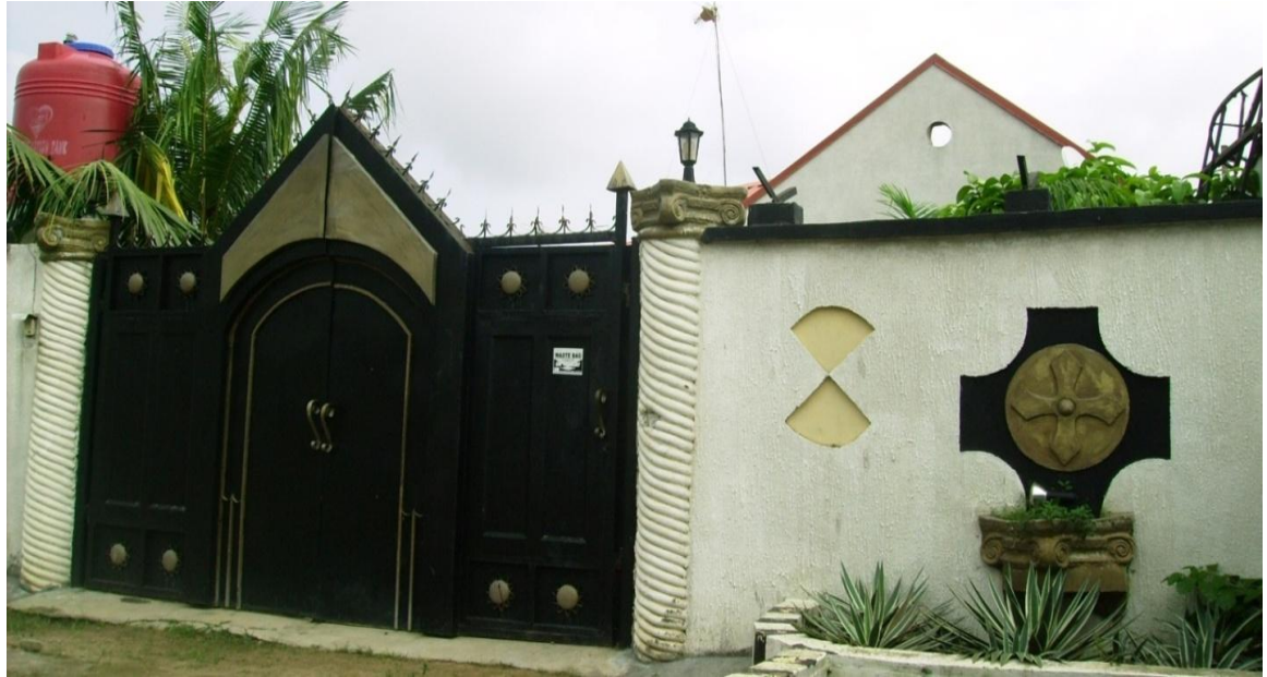
Plate 7.5: A wing of a 3-bedroom twin bungalow that has witnessed extensive transformation
