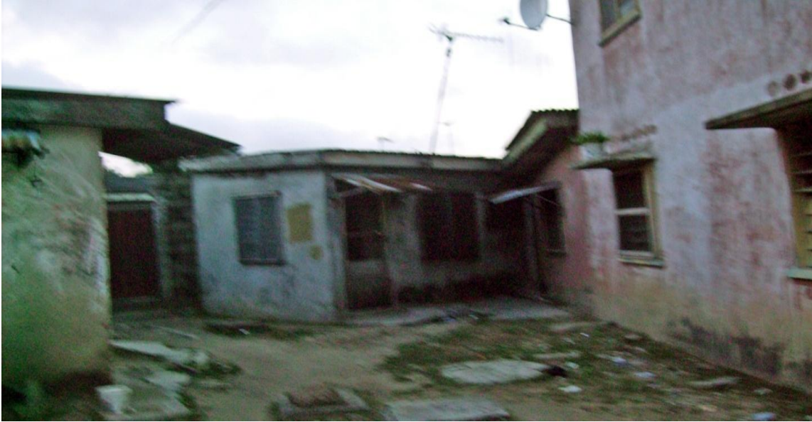
Plate 7.3: Shows Attachments Of An Illegal Structure To An Existing Building And Encroaching Into Open Space.
