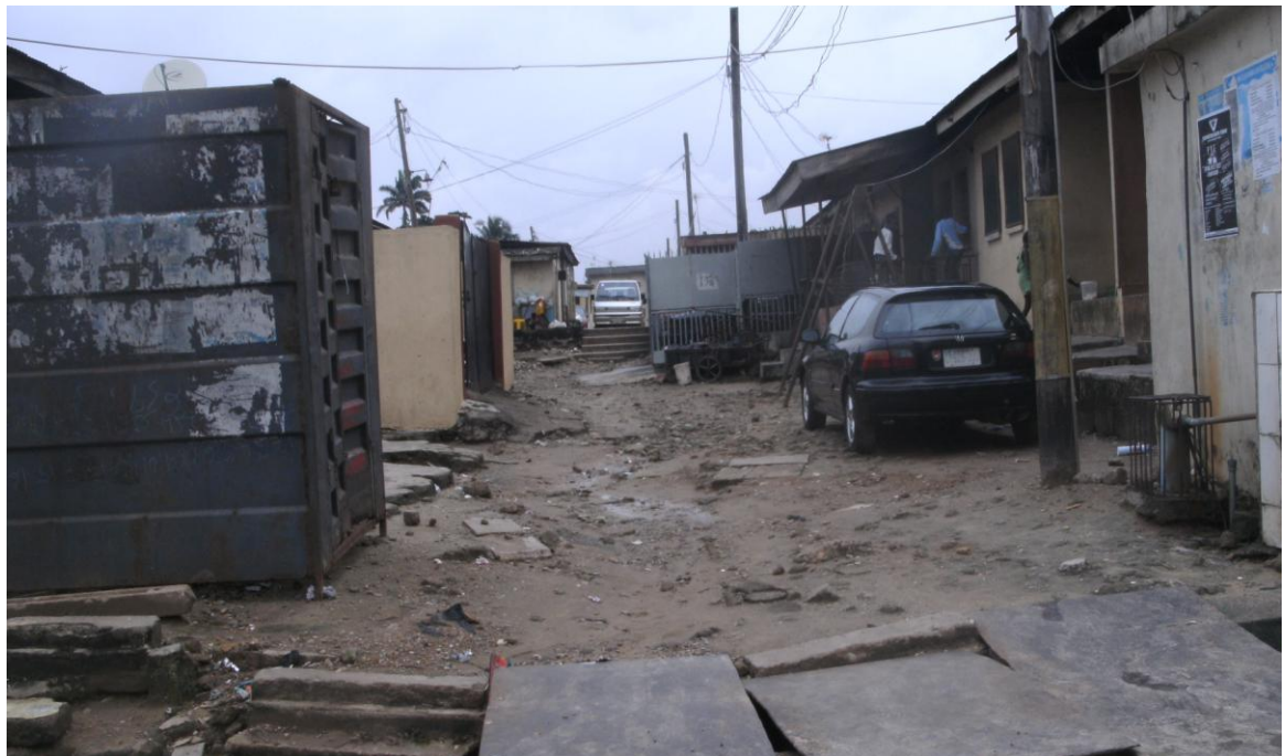
Plate 7.4: Shows An Unplanned Development And Abuse Of Building Setbacks
