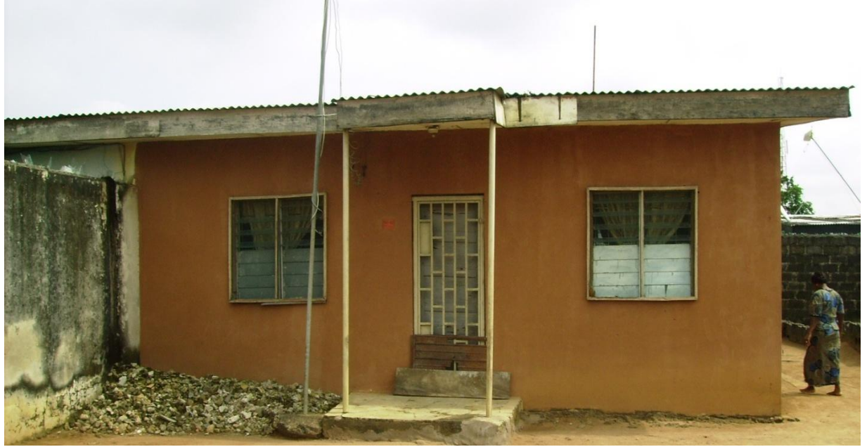
Plate 5.2: Present state of one of the few untransformed houses in Federal Low Income Estates Ipaja
