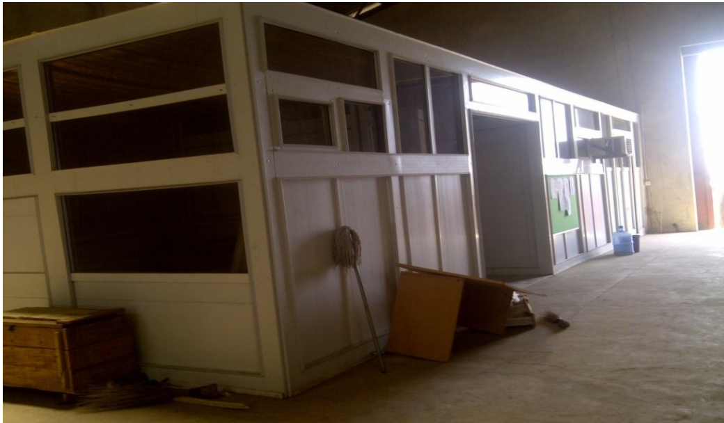
Figure 5: a complete assembled PVC structure used as an office in IBP industry, Idu yard, Abuja.
