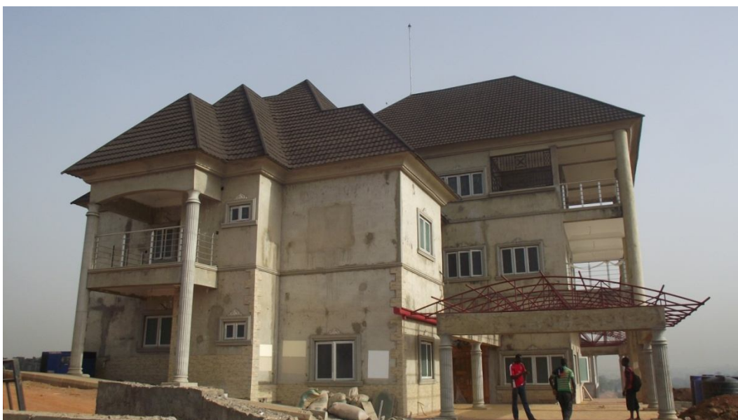
Figure 7: A Finished Building Construction in Abuja where EPS was used
