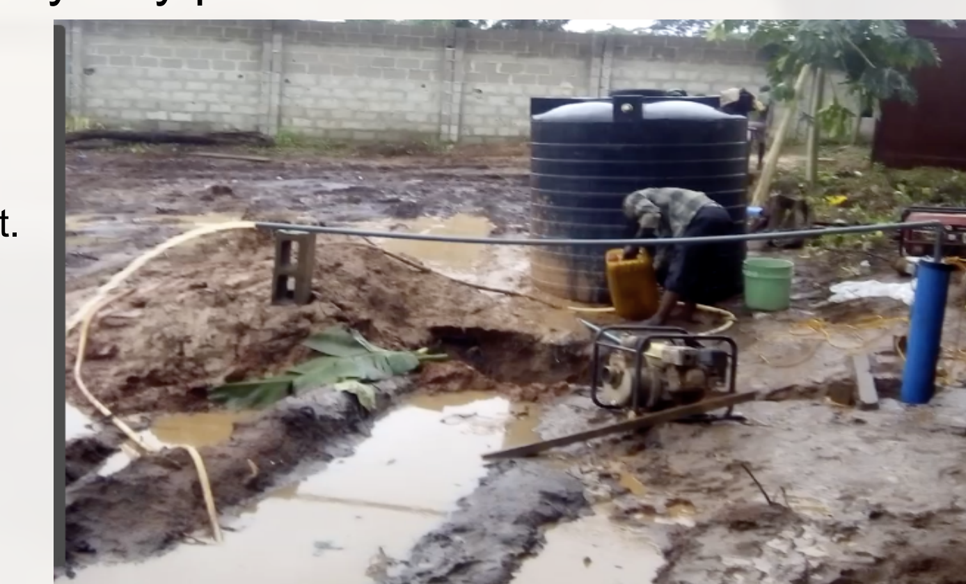
Pumping test at the location to the right.
