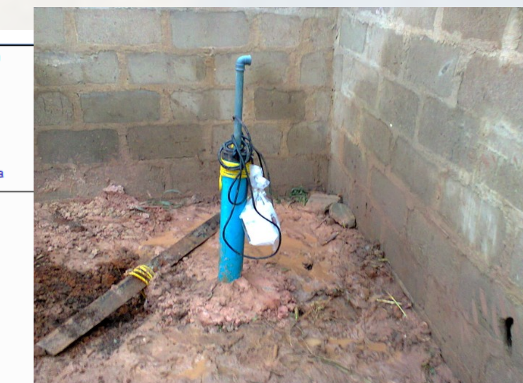
Finished bore hole
