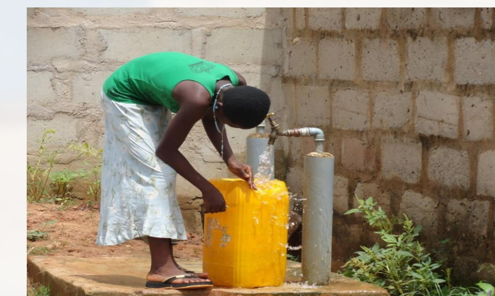
Getting freshwater from the finished borehole
