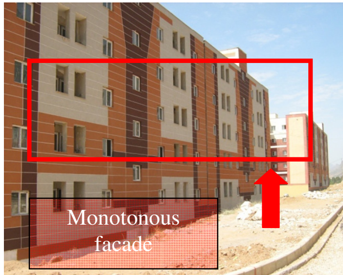
Figure 7: monotonous façade of building
