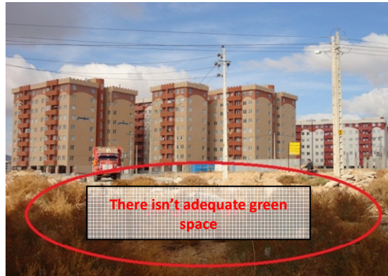
Figure 1-2-3: there isn't adequate green space
