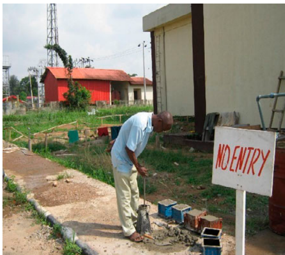
Plate 4 Casting of concrete cubes
