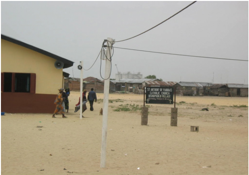
Power Distribution Line.
