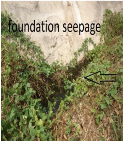
Figure 9 Foundation seepage
