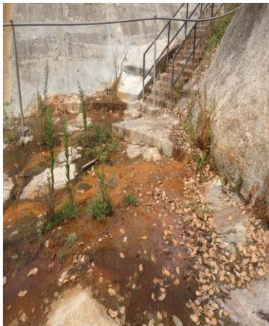
Figure 7 Seepage from the concrete/rock interface
