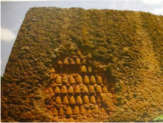
Figure 3: An Old mosque in Zaria, Northern Nigeria showing a Detail of the Tubali technique [35].
