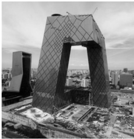
Figure 4(b): The new China Central Television headquarters building as seen in Beijing Thursday July 17, 2008. The building consists of two angled towers connected at the top to form a continuous loop of horizontal and vertical sections. The spectacular 230 meter (755 foot) building, one of Beijing's tallest, houses more than 10,000 staff. The building is one of a series of landmarks, notable for their futuristic design.
