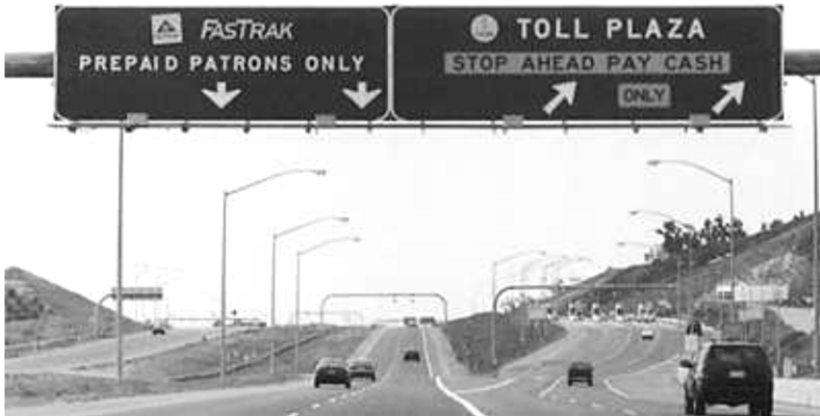
Figure 2(a): Tomato Springs Toll Plaza, just south of the CA 241 / CA 133 interchange. FasTrack is an automated toll system that requires a transponder in the car.
