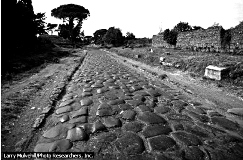
Figure 1: The cobbled Appian Way was constructed more than 2200 years ago as the primary route from Rome to Greece. Although these large lava blocks may not be the original material, the route itself has remained unchanged and in use since it was first paved.
