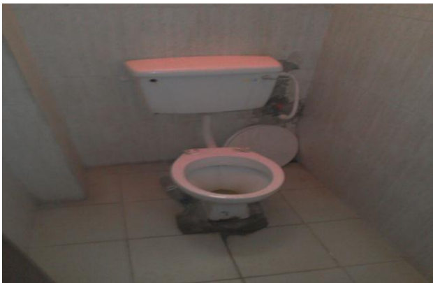
Figure 4: A typical example of toilet facility of the Museum.
